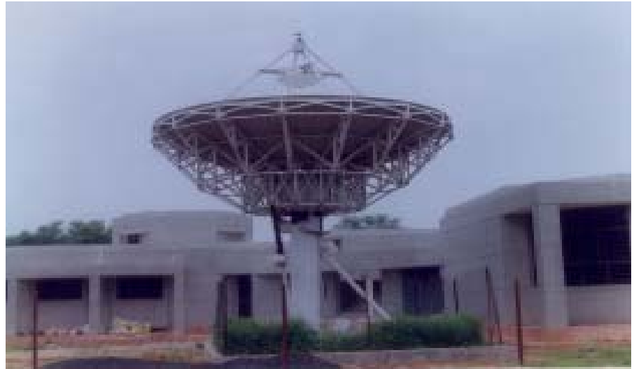
SATCOM Earth Station
