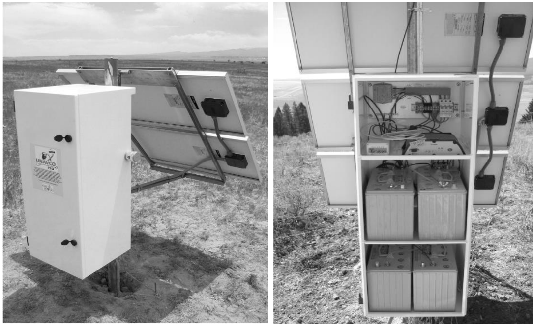
Figure 5: Enclosure with Solar Panel (Source: UNAVCO)
